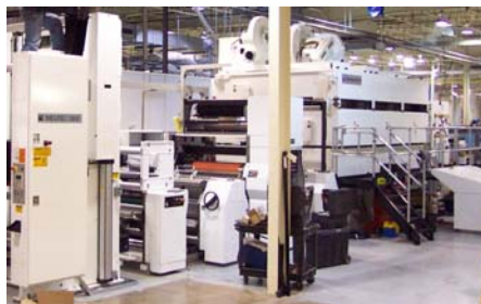
Photo of the new Timsons being installed at SBI.
